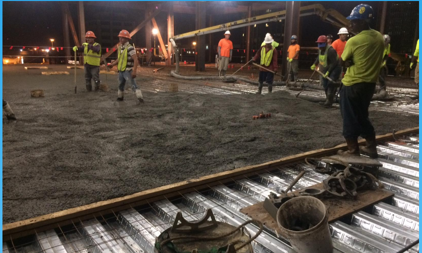
Placing concrete on metal deck 3rd floor
